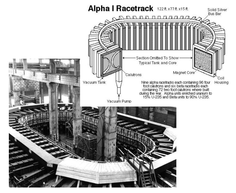
Alpha Track <u>Calutron</u> at the Y-12 Plant at Oak Ridge, Tennessee from the Manhattan Project, used for uranium enrichment by electromagnetic separation process.
